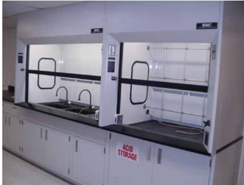
Figure 5.01 Example of horizontal sash chemical fume hoods
